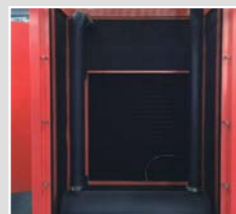
09 Internal box-type silencer –Attenuates exhaust noise in the roof and air in/outlet
