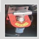
Battery isolator standard installed in the auxiliary power system of the genset, which allows disconnection for periods of inactivity without having to disconnect the battery terminals.
